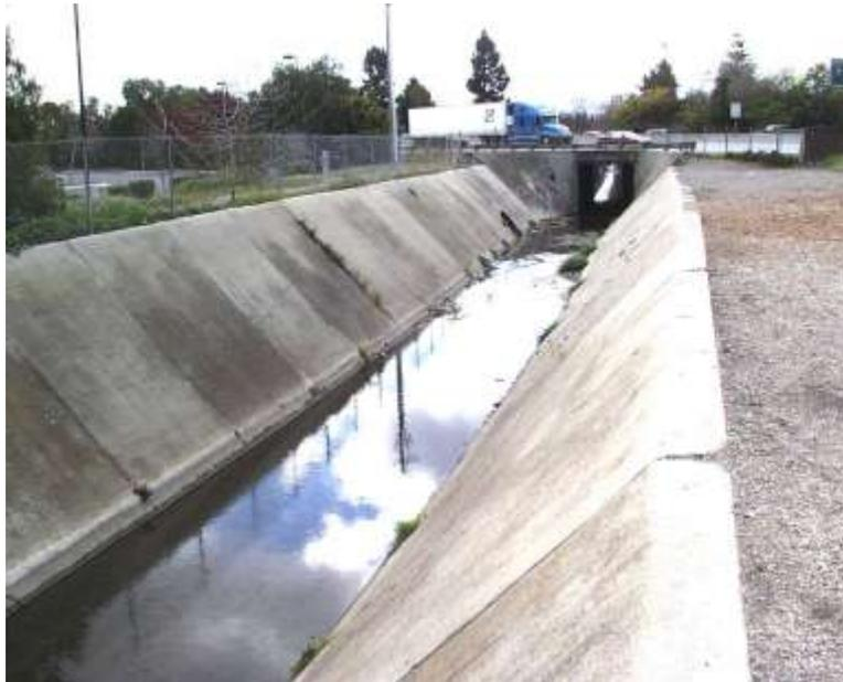
**Figure 7-2(b). Permanente Creek looking upstream at Hwy 101. Concreted steep banks were constructed in early 1960's to support urban development.**
