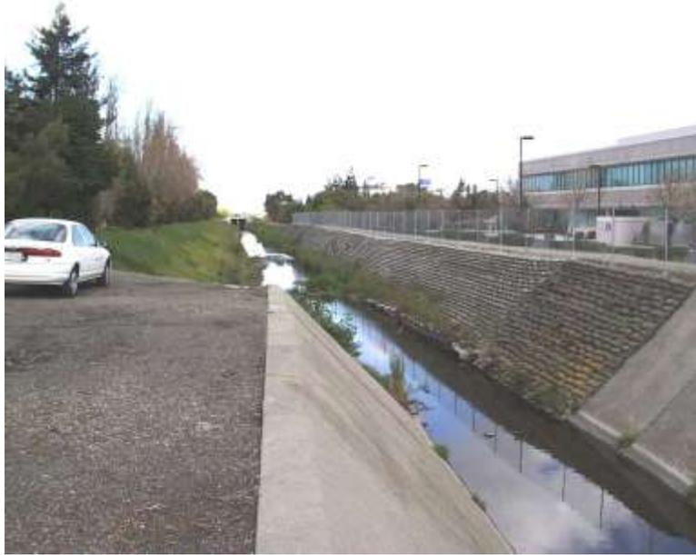
**Figure 1-2(a). Permanente Creek looking downstream from Hwy 101 towards Charleston. Concrete and concrete sacks line the channel to support steep channel banks following urbanization. Construction work completed in 1963.**
