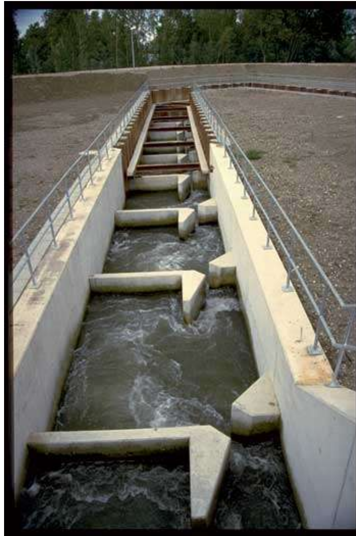
Figure 6-10. Vertical Slot Fishway [From FAO Fisheries Department]
