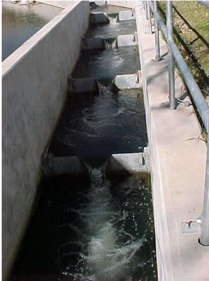
Figure 6-9. Compound Weir Shape at Masson Dam on Guadalupe Creek
