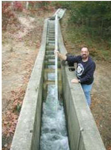
Figure 6-12. Denil Fishway in Operation (From Massachusetts Dept. of Marine Fisheries)
